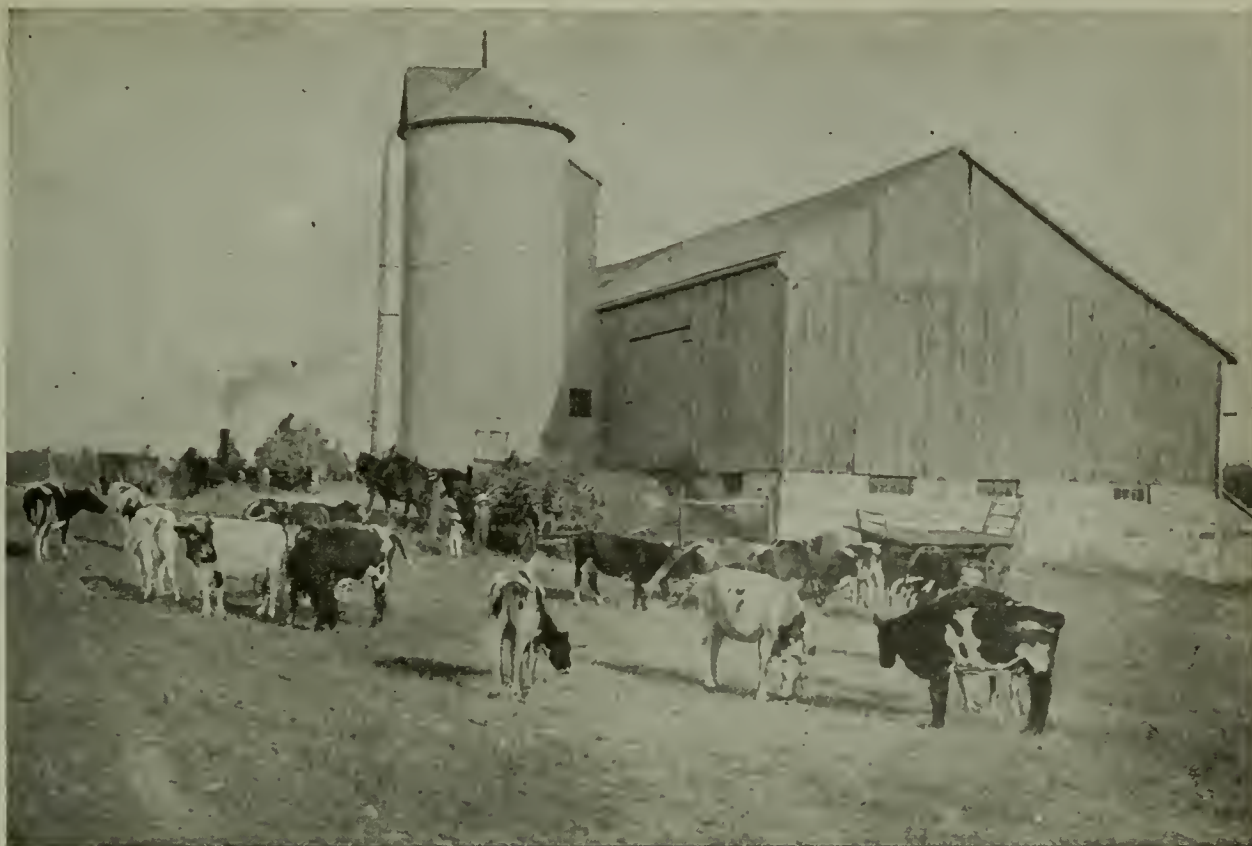
A tower, called a silo, in which green fodder is stored for the winter by compressing it while still green, and keeping it covered from the air. The fodder thus preserved is called ensilage, or silage.
